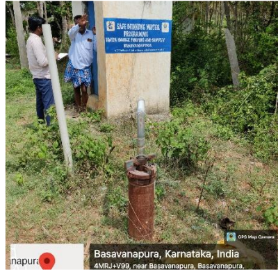
Pipeline extension motor in Basavanapura
